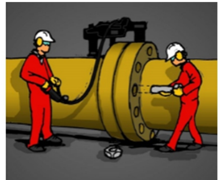
Powermaster flange alignment method
